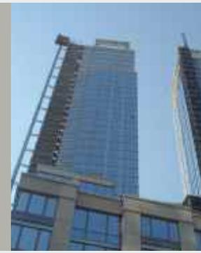
sides of the load bearing columns to protect against the influence of wind. Together with the architects and structural engineers, Getzner prepared detailed load distribution plans, in which the loads on each of 350 bearing points was precisely determined. The ground floor was constructed using support beams and in the first floor, the isolation is recessed in the ceiling. The new construction method with T-beams helps minimize the build-up height.
